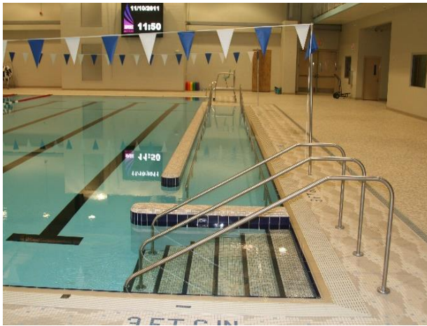
Permanent Built in Ramp and Stairs
