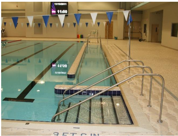
Permanent Built in Ramp and Stairs
